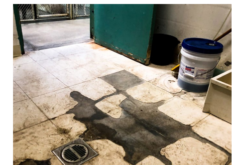
Flooring cracked and torn
